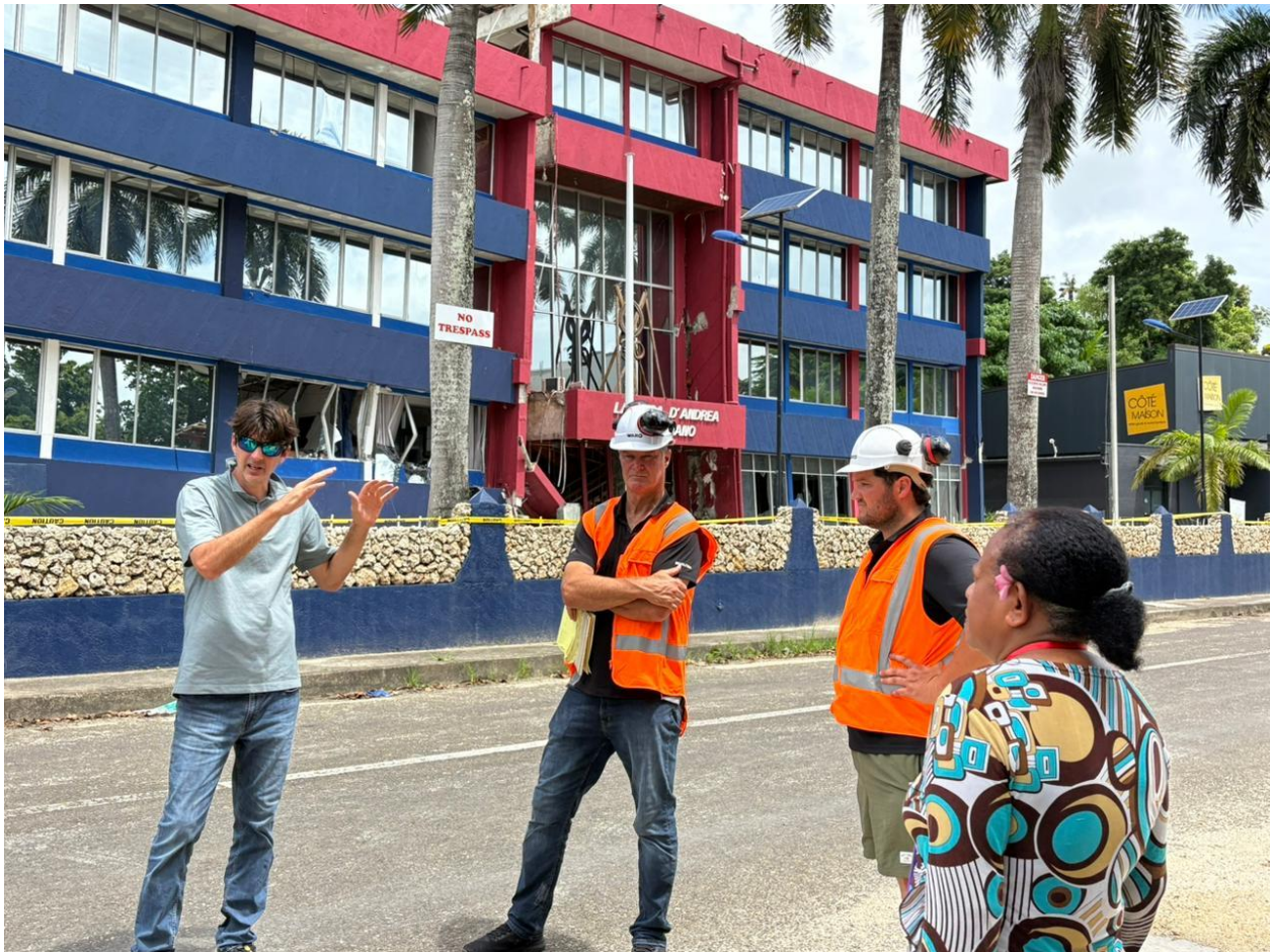
DG PMO - CheroI ianna Ala getting an update report from Pierre Brunet Enterprise General and NZ contractors on the planned demolition of Chantilly's On The Bay and La Casa De Andrea in Port-Vila - 08 January 2025
